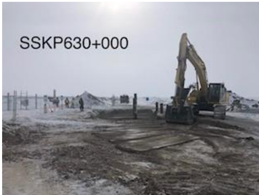
Backfill complete at MLBV 16
