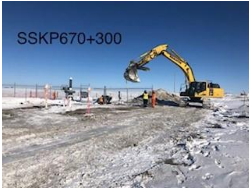
Facilities crew installing fence at MLBV15
