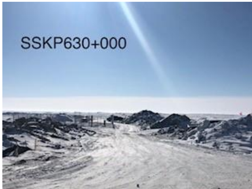
Facilities construction sweep crew - line locating
